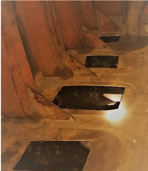
Openings Cut to Remove Zincs
