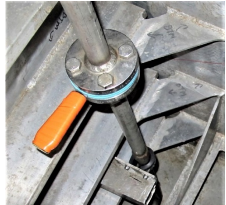
Putty Knife "Blind" in a Flange
