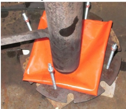
Jacking Plate with Gasket Seal
